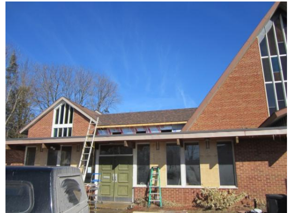
... raising the roof for accessibility
